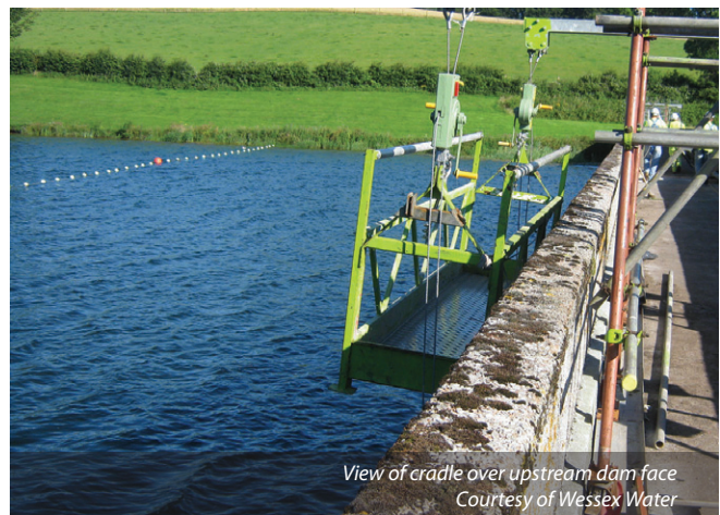
View of access gantry to underside of bridge deck from the bridge deck - Courtesy of Wessex Water
