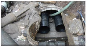
1,050mm culvert with lower UV liner in place receiving flow and 2 (No.) HDPE surcharge relief pipes above awaiting grouting. Note the pump bypass pipe to the left threaded through an adjacent EA culvert which had been transferring flow downstream prior to UV lining Courtesy of WECS
