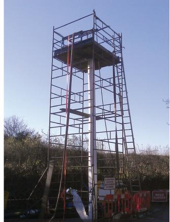
Eversion towers from which the lining is launched and the height is calculated to ensure enough head of water to drive the liner through the sewer and overcome any frictional losses - Courtesy of WECS
