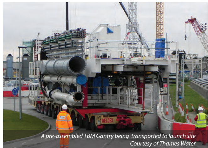
View of temporary TBM Gantry in operation Courtesy of Thames Water
