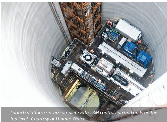
View of launch platform installation nearly complete - Courtesy of Thames Water
