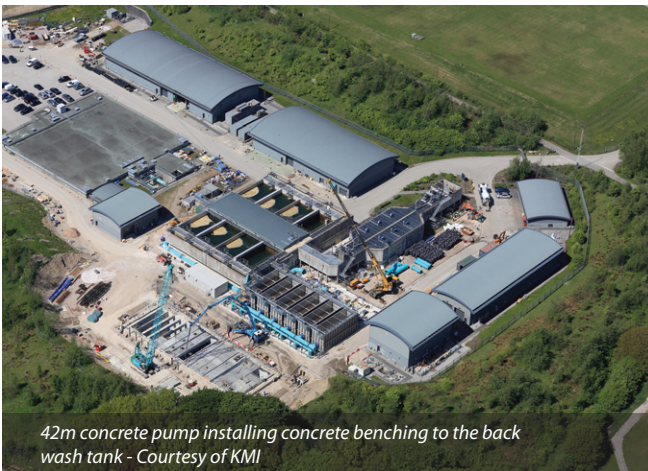
Backwash tank before roof beams/slabs have been installed Courtesy of KMI
