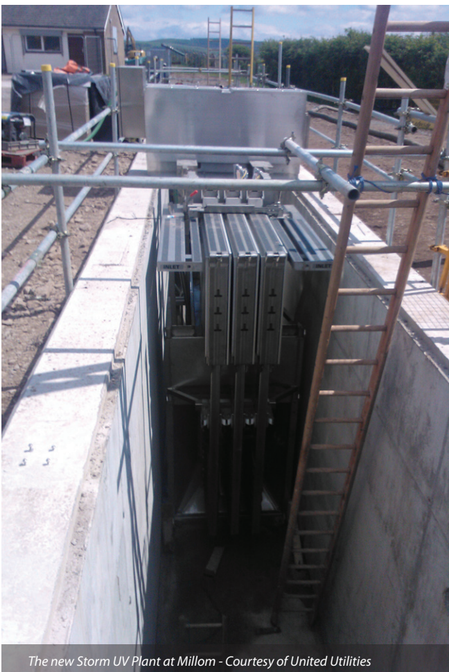
Storm UV plant at the fabrication - Courtesy of Trojan
