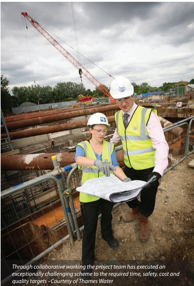
Final settlement tank base pour Courtesy of Thames Water
