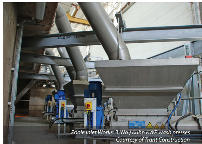
Inlet screens installation nearing completion Courtesy of Trant Construction Ltd
