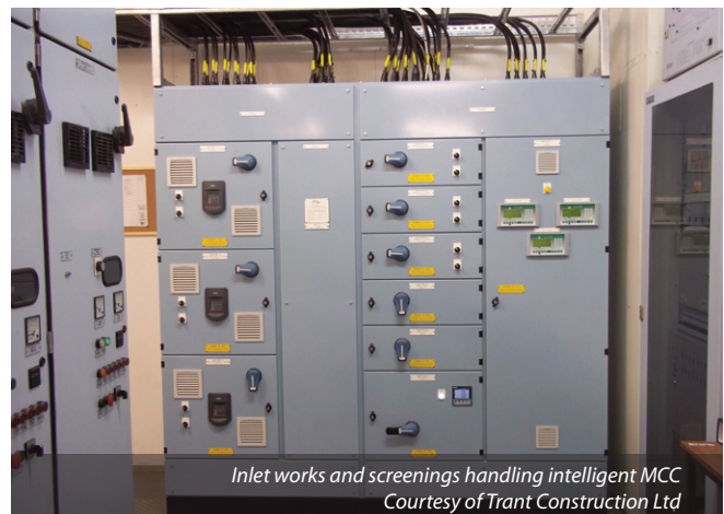
Poole Inlet Works - CF200 fine screen installation Courtesy of Trant Construction Ltd
