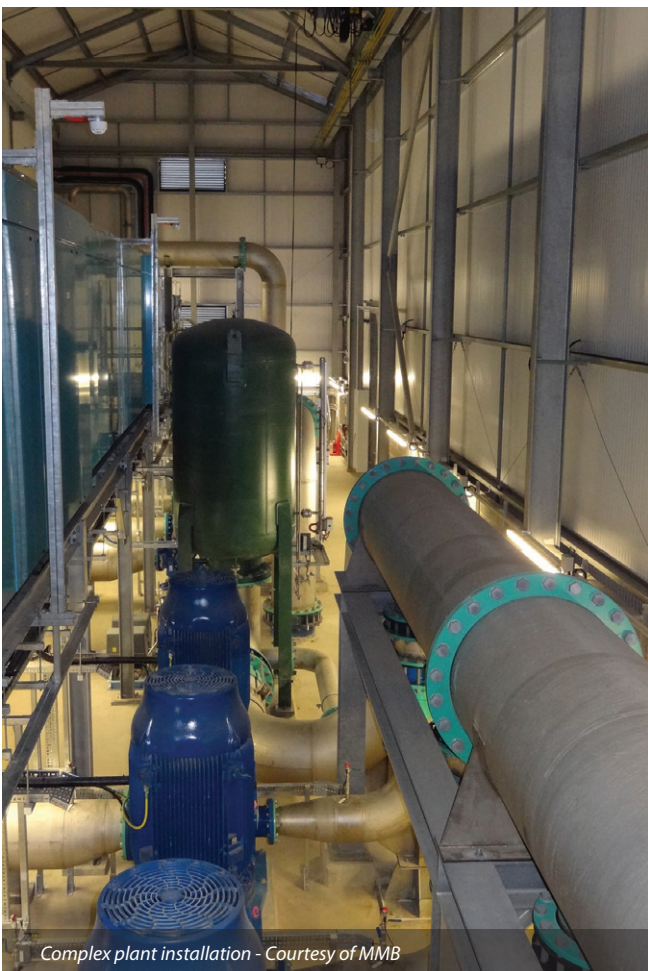
Construction of the new building at Rivelin WTW - Courtesy of MMB
