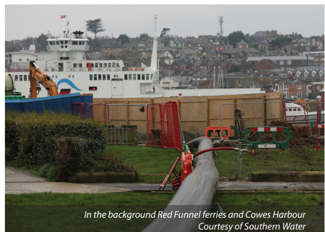
The reception pit at East Cowes - Courtesy of Southern Water
