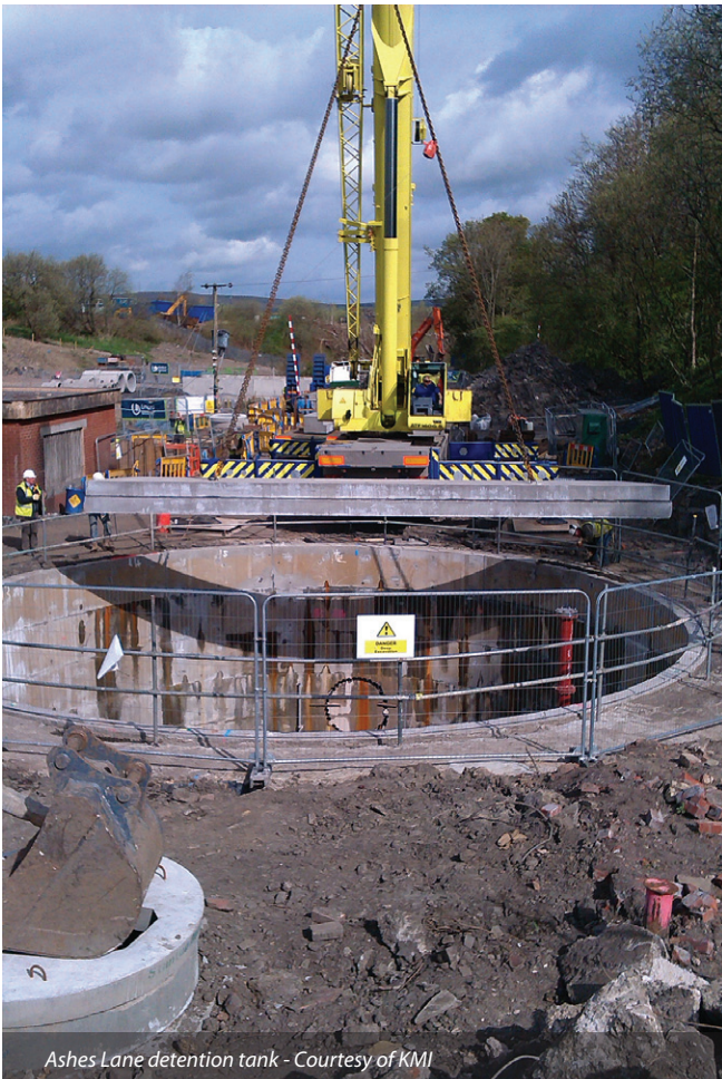
Middleton Road pipeline auger bore - Courtesy of KMI
