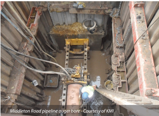
Middleton Road pipeline auger bore - Courtesy of KMI
