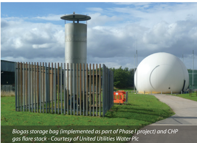
One cell of ASP1 (refurbished) Courtesy of United Utilities Water Plc
