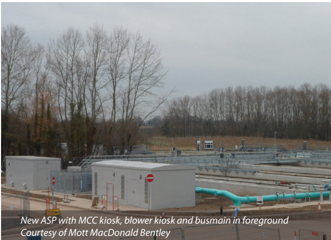
Anaerobic/anoxic tank Courtesy of Mott MacDonald Bentley
