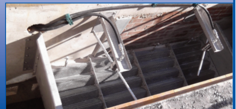
*Hydrok stainless steel wedge wire profiles utilised in all Hydrok CSO screens
