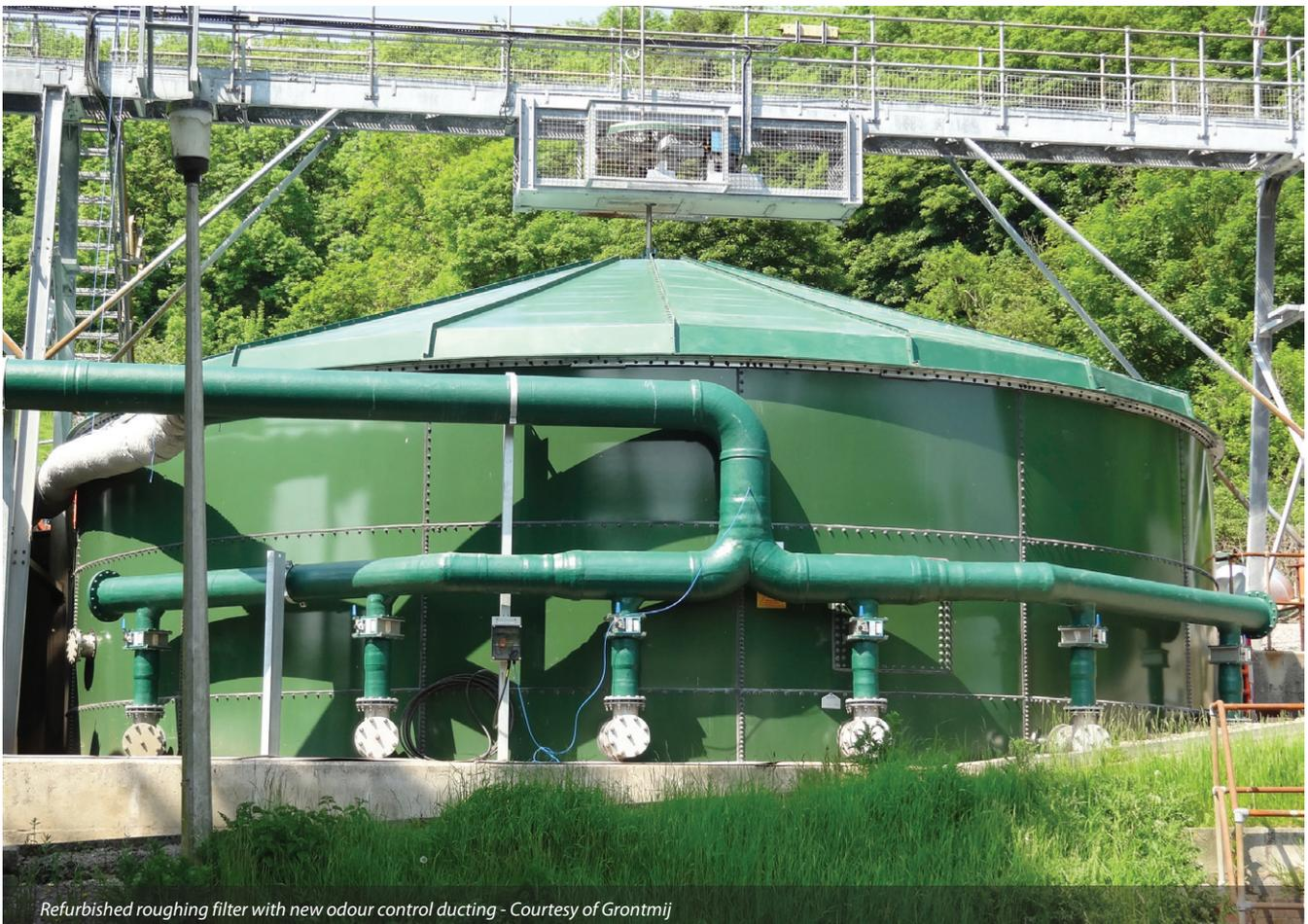
Refurbished roughing filter with new odour control ducting - Courtesy of Grontmij
