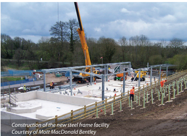
Concrete slab construction Courtesy of Mott MacDonald Bentley
