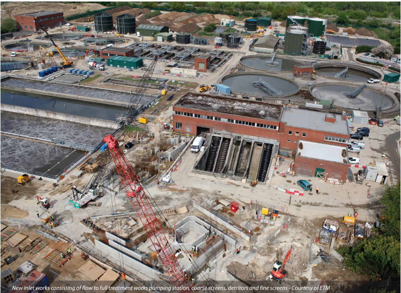
New inlet works consisting of flow to full treatment works pumping station, coarse screens, detritors and fine screens - Courtesy of ETM
