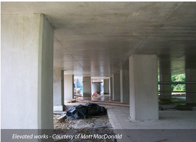
View of elevated channels - Courtesy of Mott MacDonald
