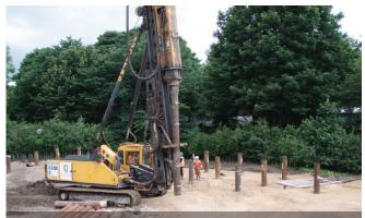
Advance piling: driving steel piles for the elevated inlet works. Crushed concrete working platform subsequently incorporated into the permanent works - Courtesy of Mott MacDon
