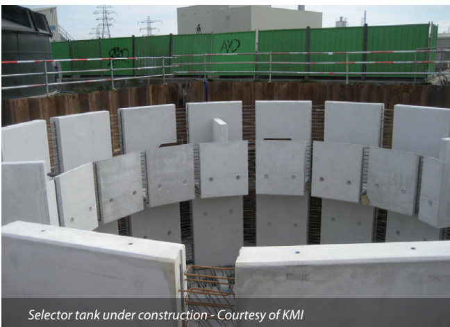
Placing selector tank wall panels - Courtesy of KMI
