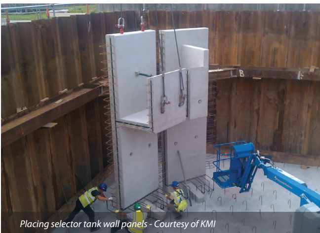
Detention tanks under construction - Courtesy of KMI
