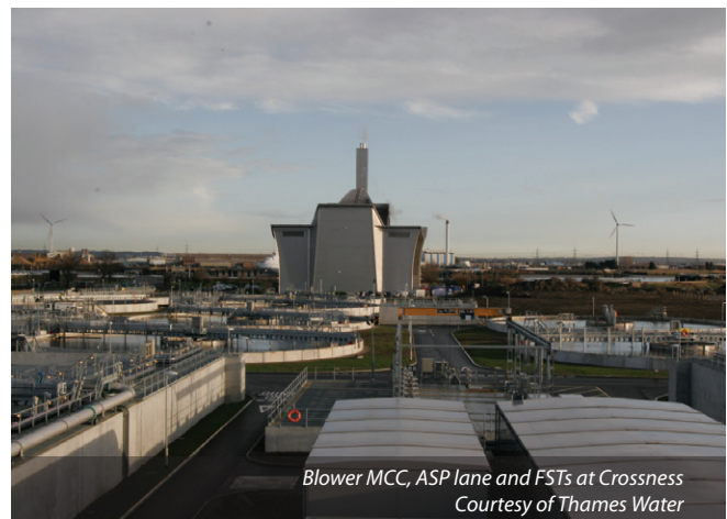
Western aeration lane (ASP) and final settlement tanks (FST) at Crossness - Courtesy of Thames Water
