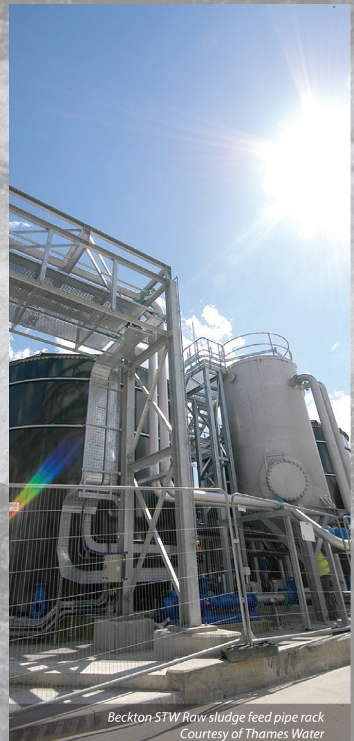
Beckton STW Raw sludge high energy mixing and storage - Courtesy of Thames Water
