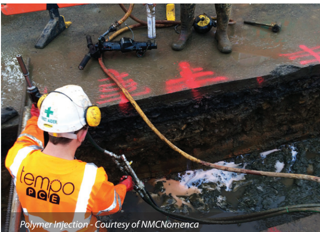
Material prior to excavation - Courtesy of NMCNomenca
