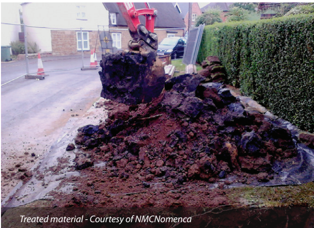
Polymer Injection Trial in Church Street - Courtesy of NMCNomenca
