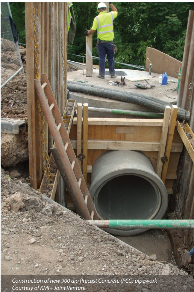
View through inlet channel into detention tank - Courtesy of KMI+ JV
