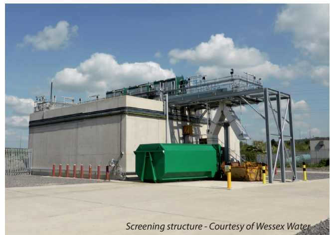
New Coarse Screening facility at Bristol STW - Courtesy of Wessex Water
