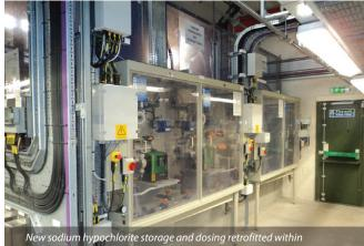
New sodium hypochlorite storage and dosing retrofitted within the existing chemical building - Courtesy of KMI+
