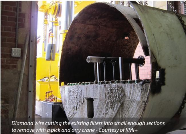
Diamond wire cutting the existing filters into small enough sections to remove with a pick and pry crane - Courtesy of KMI+
