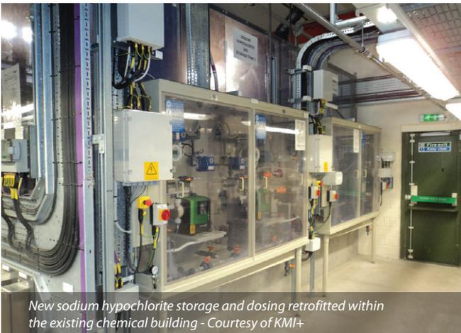
New sodium hypochlorite storage and dosing retrofitted within the existing chemical building - Courtesy of KMI+
