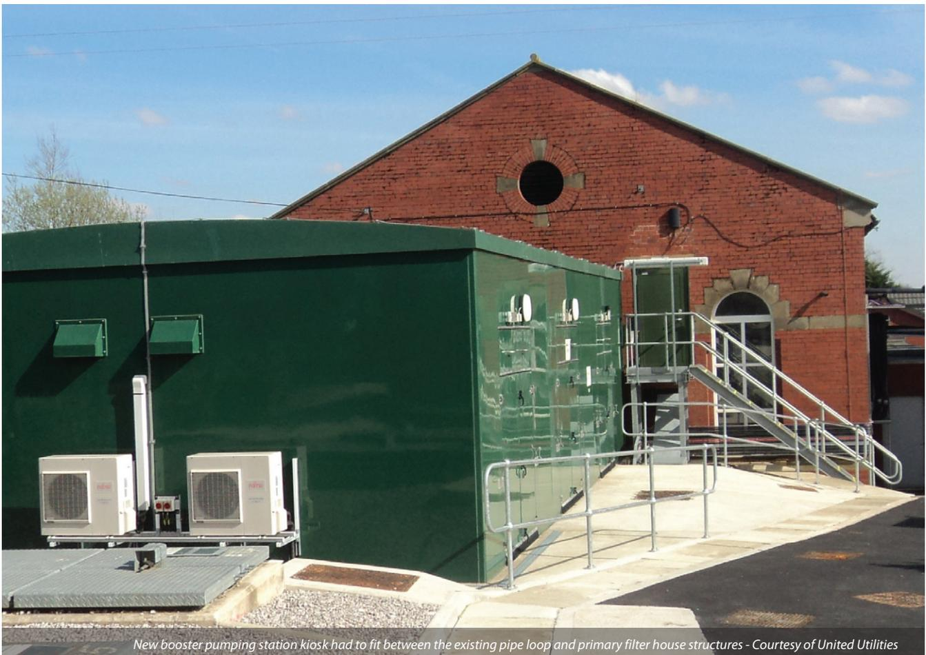
*New booster pumping station kiosk had to fit between the existing pipe loop and primary filter house structures - Courtesy of United Utilities*
