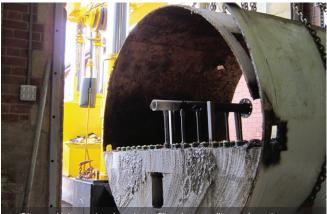
Diamond wire cutting the existing filters into small enough sections to remove with a pick and arry crane - Courtesy of KMI+
