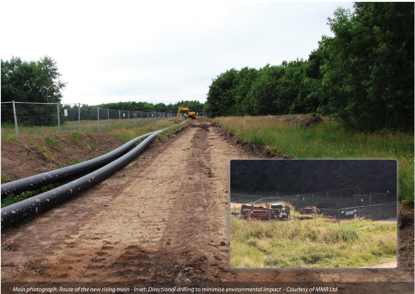
Main photograph: Route of the new rising main - Inset: Directional drilling to minimise environmental impact - Courtesy of MMB Ltd
