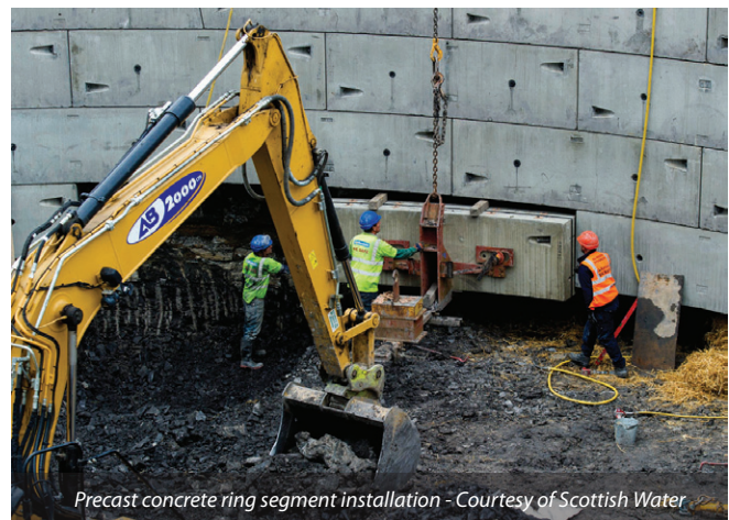
3000m 3 storage tank underway by Barhale Courtesy of Scottish Water
