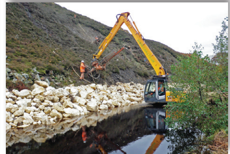
Soil nailing and netting to safeguard assets
