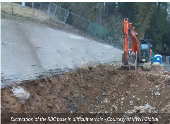
The original plant had no vehicle access and there was no land available for additional assets - Courtesy of MWH Global
