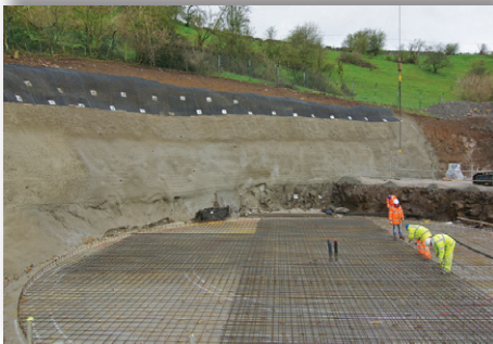
Anchoring and sprayed concrete to support tank excavation
