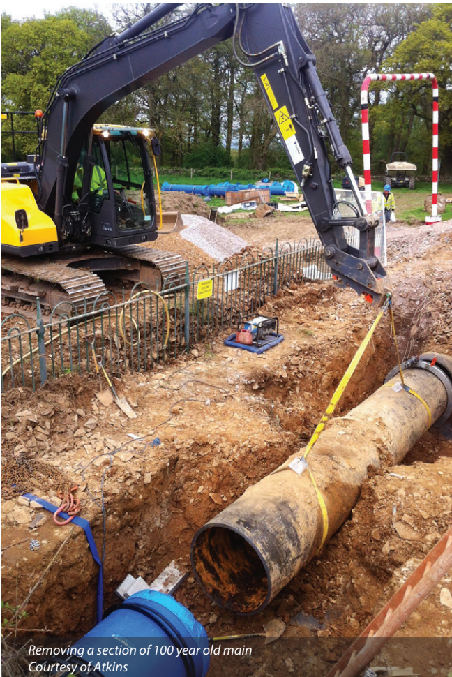
Preparing to drill a large diameter under pressure tapping Courtesy Laing O'Rourke
