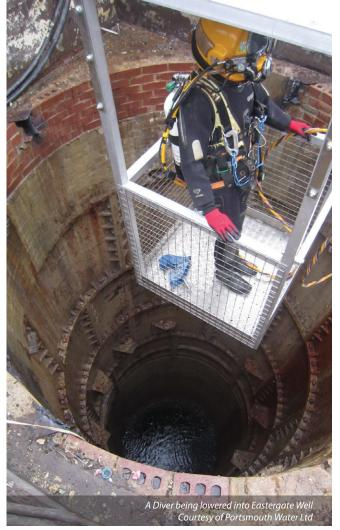
the borehole there are numerous fissures which yield raw water from the South Downs. The well and borehole was originally sunk in 1893, the well measuring 2.4m in diameter and 25m in depth. The borehole was reamed out in 1993 to a diameter of 1.2m and its current depth is 65m below ground level. The widening of the borehole increased the sources total yield which allowed it to cope with the rising local population.
