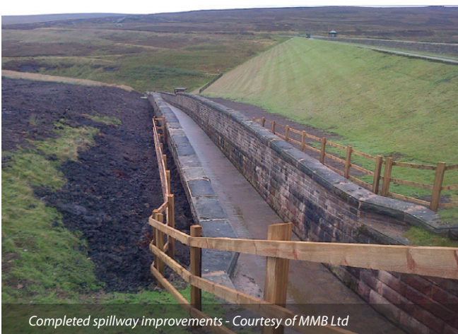
Culvert with porcupine block downstream headwall Courtesy of MMB Ltd
