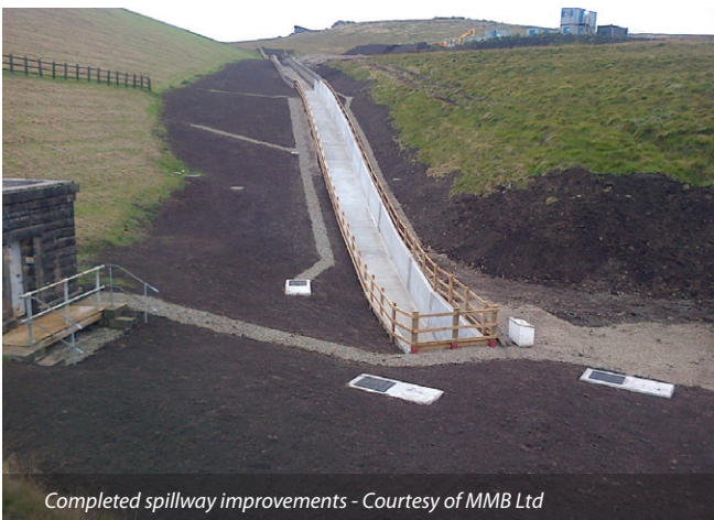
Completed spillway improvements - Courtesy of MMB Ltd
