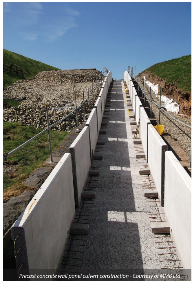
Challenging Site Logistics - Courtesy of MMB Ltd
