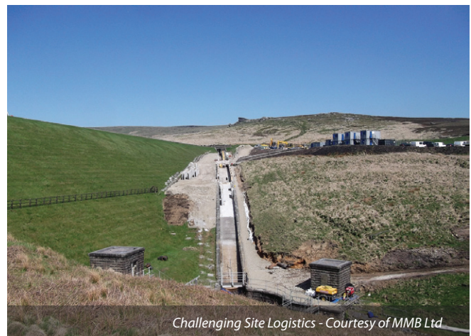
Spillway improvement works at Gorple Upper Reservoir Courtesy of MMB Ltd
