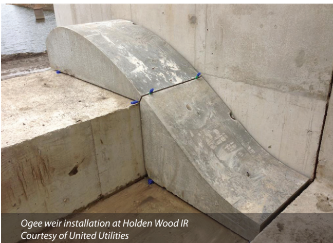
Diamond chainsaw and a large diameter saw cut through Holden Wood IR crest - Courtesy of United Utilities
