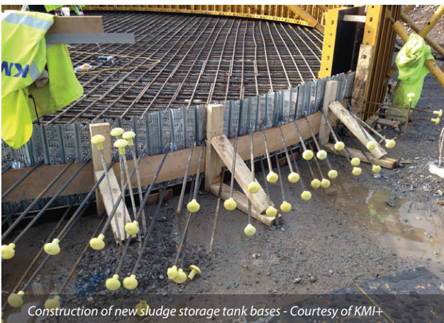
Construction of new sludge storage tank bases - Courtesy of KMI+
