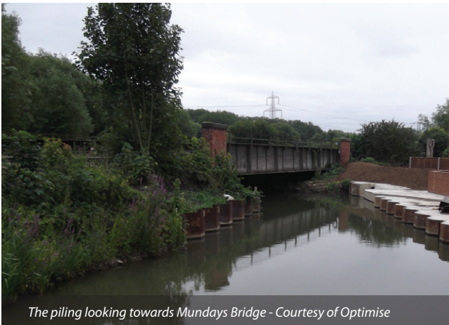
Hinksey Drain close to Munday's Railway Bridge prior to construction Courtesy of Optimise
