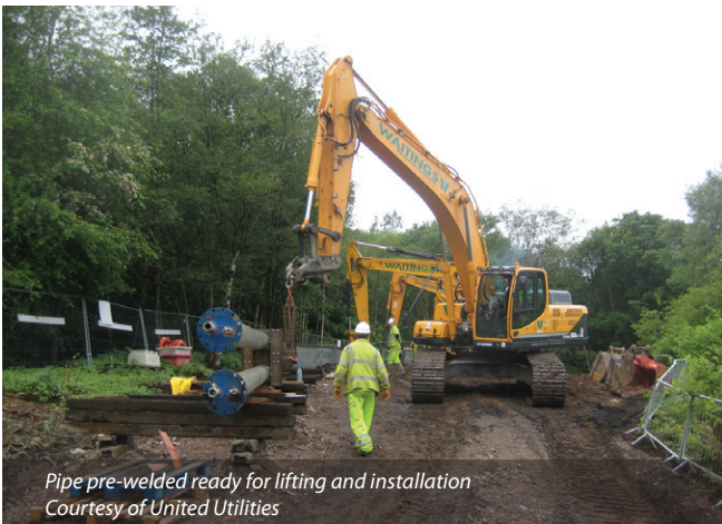
Pipe crossing trench prepared - Courtesy of United Utilities
