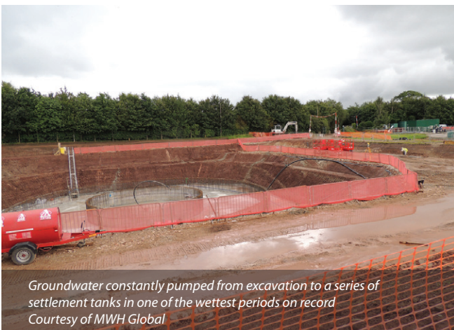
Innovative design of combined oxidation ditch and FST reduced land take and shortened the construction programme - Courtesy of MWH Global
