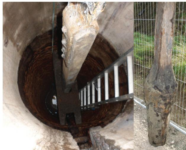
Figure 2: Neptune shaft and original wooden plug - Courtesy of CRT
