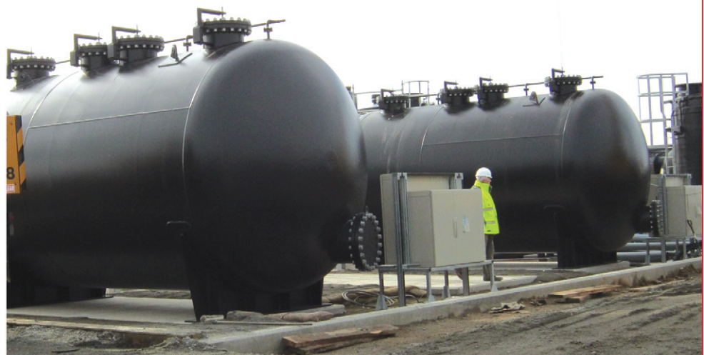
GAC & Pressure Filter Vessels used in Guernsey Airport Water Treatment Facility Project (2012) DESIGNED & MANUFACTURED BY PRESSVESS
