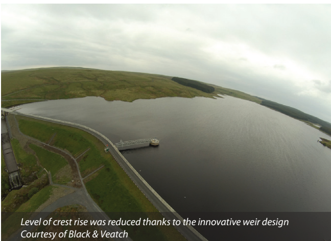
Design of the PK weirs was developed with ease of construction a significant consideration - Courtesy of Black & Veatch
