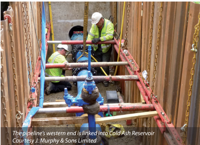
The pipeline's T-connection into its water supply source near Tilehurst Reservoir - Courtesy J. Murphy & Sons Limited
