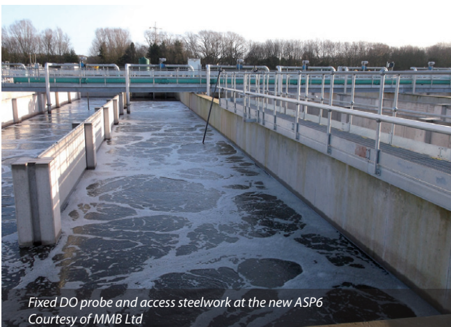
New ASP6 showing in-situ structural walls and precast baffle walls Courtesy of MMB Ltd
