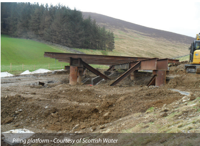
Temporary working platform - Courtesy of Scottish Water
