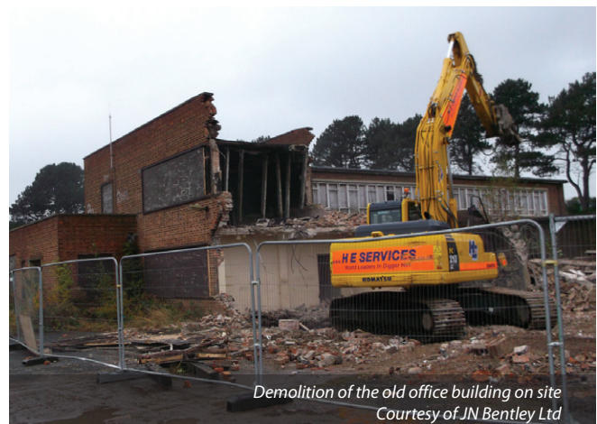
On site recycling of demolition material - Courtesy of JN Bentley Ltd
