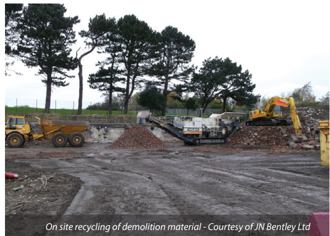
Tank wall demolition - Courtesy of JN Bentley Ltd
