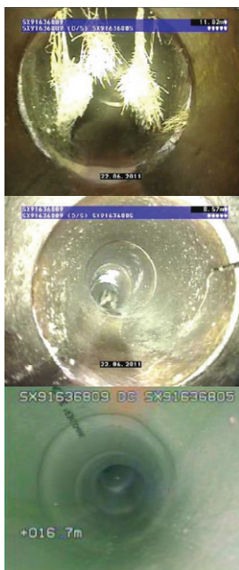
Photographs illustrating the pre-condition pipeline and post-lining improvement following installation of the Brawoliner 3D - Courtesy of BBUSL & Exjet
