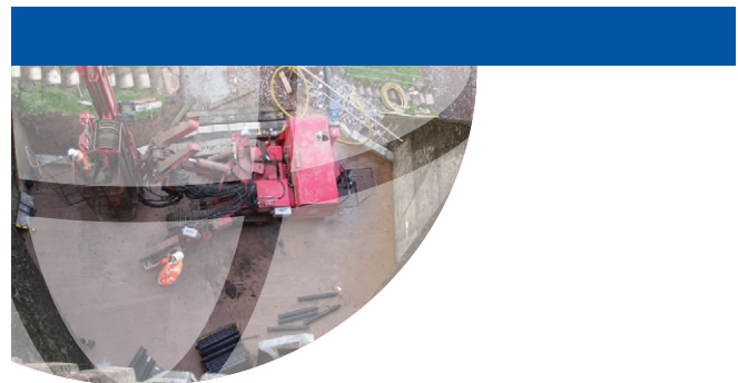
Drill rig - Courtesy of South West Water
