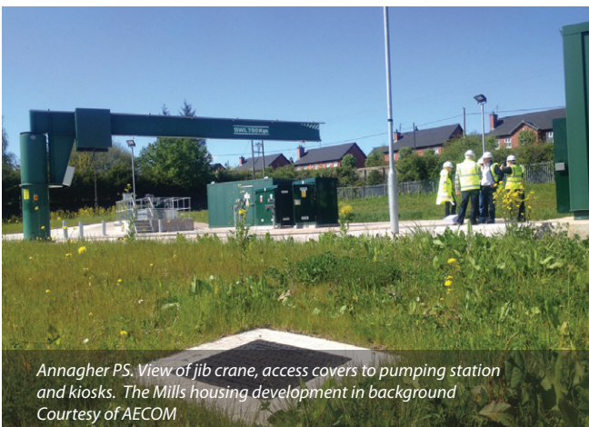
MEICA installation and commissioning - Courtesy of AECOM
