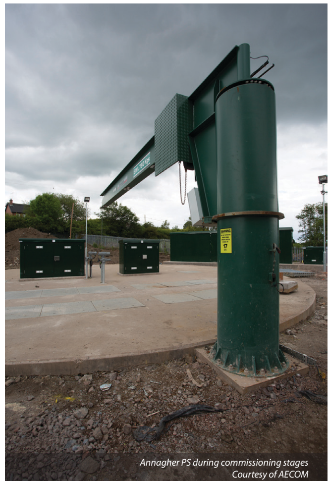
Construction of pipelines to Annagher PS. Trench 'well pointing' dewatering system - Courtesy of AECOM
