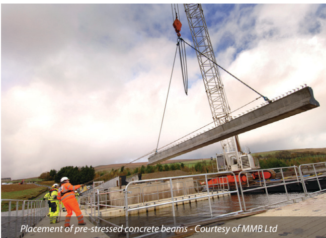
Floating pontoons with edge protection for safe access Courtesy of Mott MacDonald Bentley Ltd
