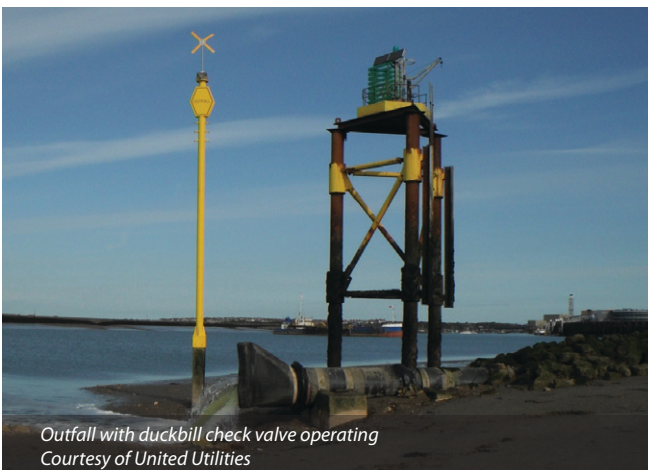
Connection to existing outfall station - Courtesy of United Utilities
