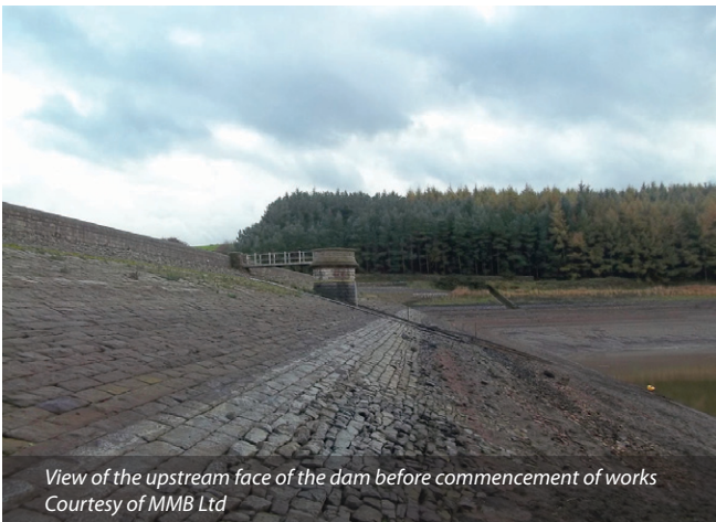
Spillway at Beaver Dyke - Courtesy of MMB Ltd
