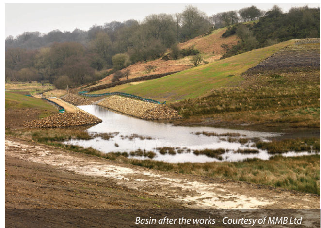
Completed discontinuance channel looking upstream Courtesy of MMB Ltd
