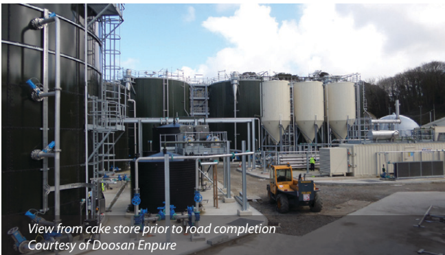
The early stages of base construction - Courtesy of Doosan Enpure
